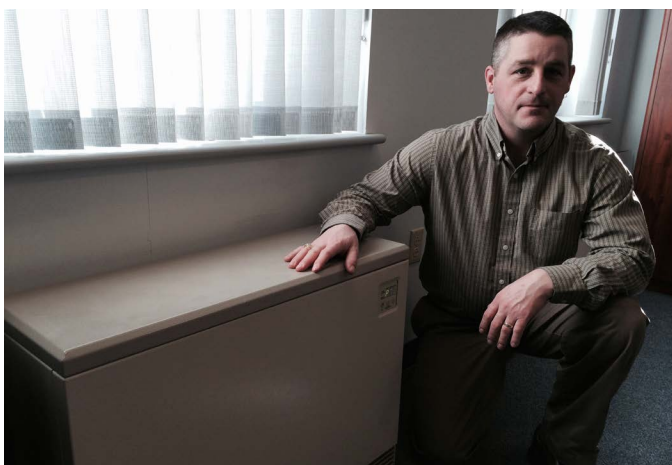
David Wood, CMLP’s general manager, with a Steffes heater. The unit is full of ceramic blocks that are heated with electricity overnight and warm his office by day.
